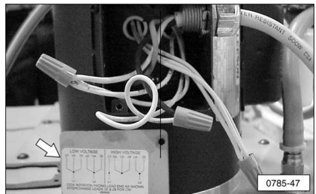
Illustration 4. Use Wiring Diagram On Inside Of Motor Cover.
